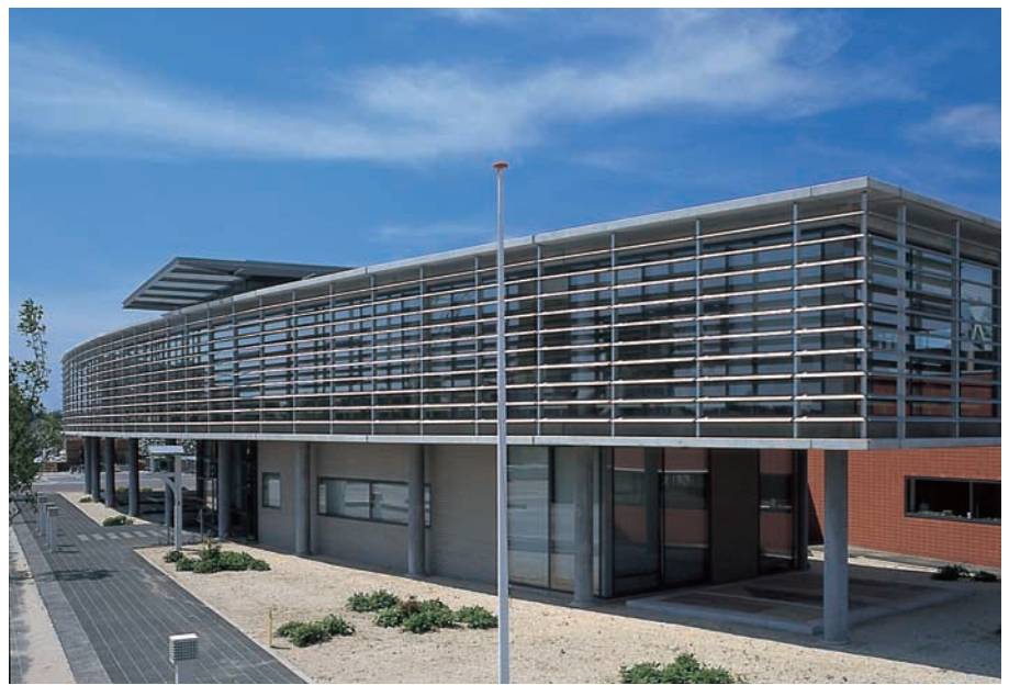
Material centre & Omegam, the Netherlands
