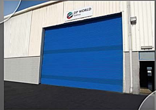
DPWorld - Roller Shutter Door - Sokhna Port
